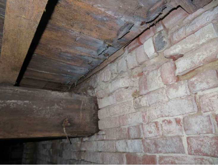
STRUCTURAL SCOPE D: REPAIR CRACKS AT BRICK MASONRY ADJACENT TO ROOF OVERHANG BRACKETS
