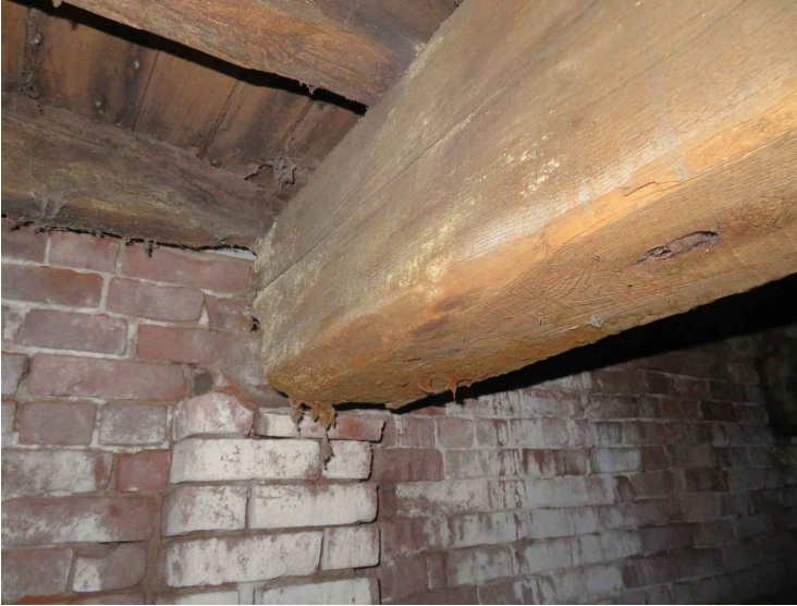
STRUCTURAL SCOPE B - PHOTOS
