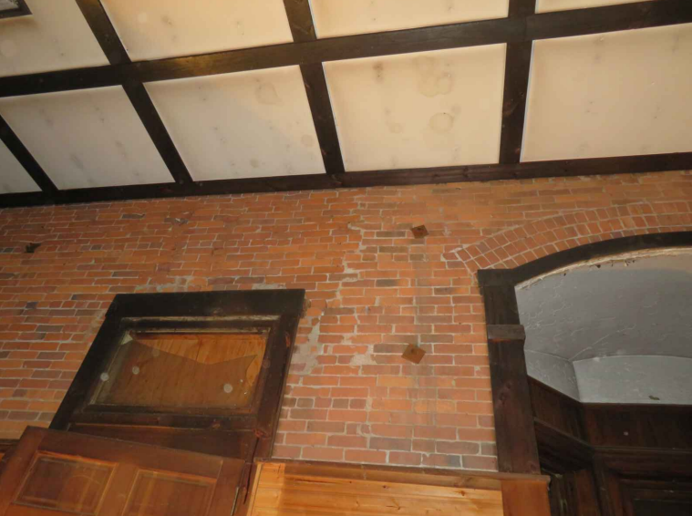
AT EAST WALL NEAR TRUSS 5
