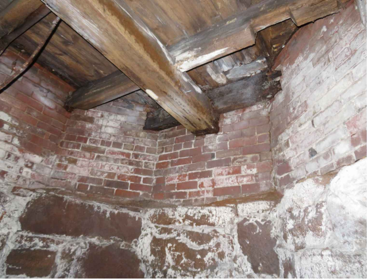
STRUCTURAL SCOPE D: REPAIR CRACKS AT BRICK MASONRY ADJACENT TO ROOF OVERHANG BRACKETS
