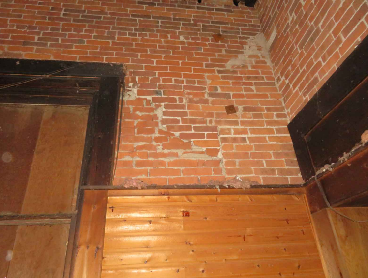
AT WEST WALL NEAR TRUSS 3
