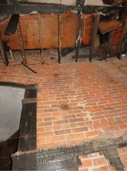
AT WEST WALL NEAR TRUSS 5
