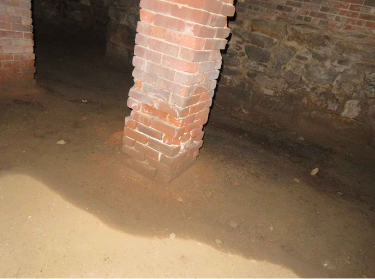
STRUCTURAL SCOPE A: REMOVE BRICK PIERS AFTER INSTALLATION OF NEW COLUMNS
