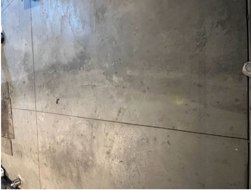
Photo 1 of Hughes concrete garage floor without cracks taken 10/5/22.
