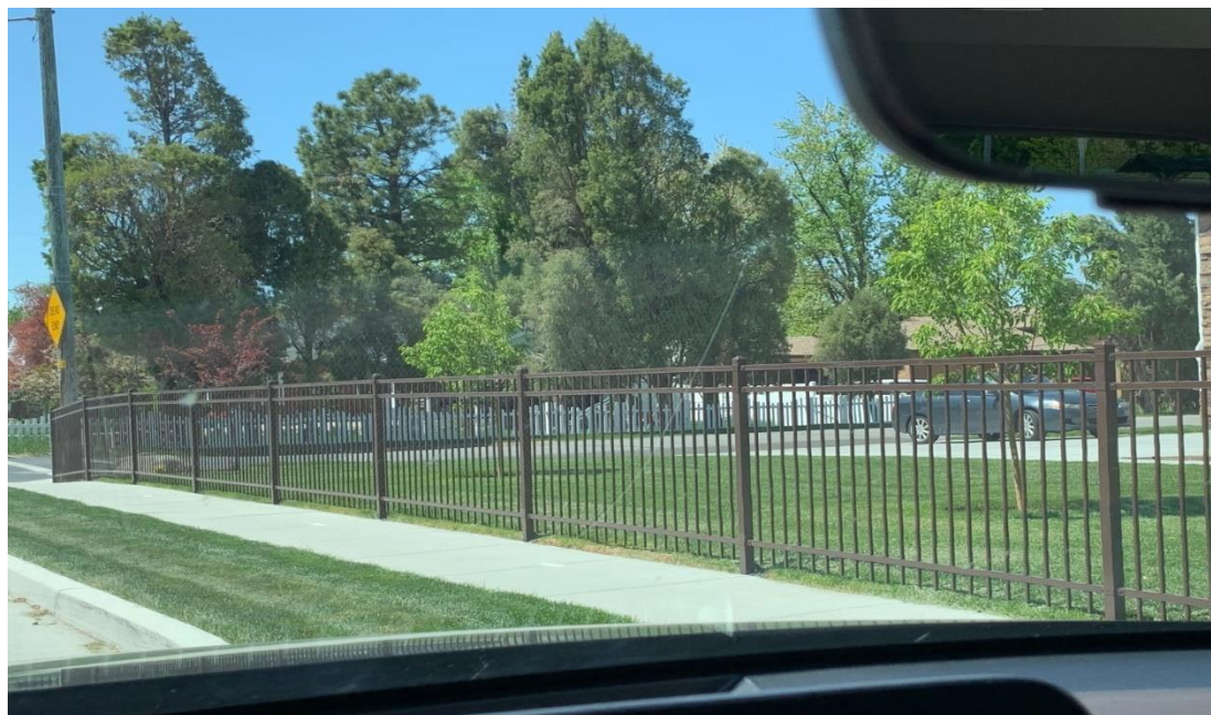
EXAMPLE OF OPEN FENCING
