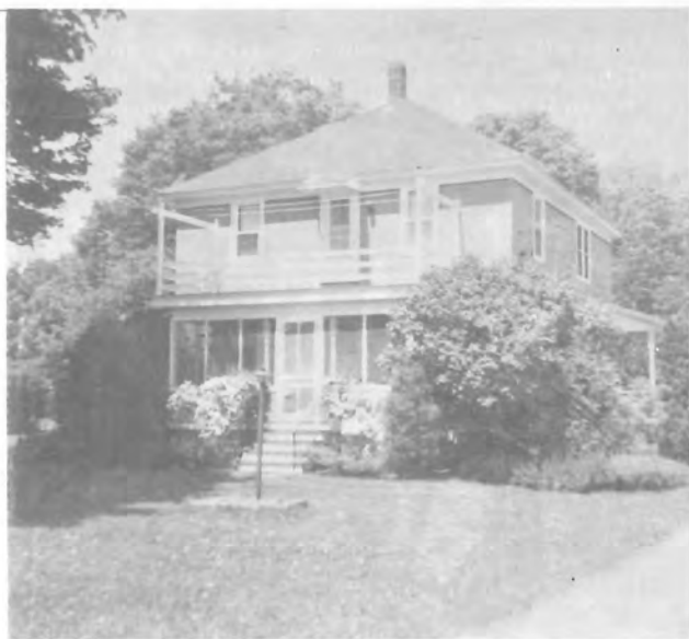
Quarry rooming house. Now the Edward Brandenberg home.
