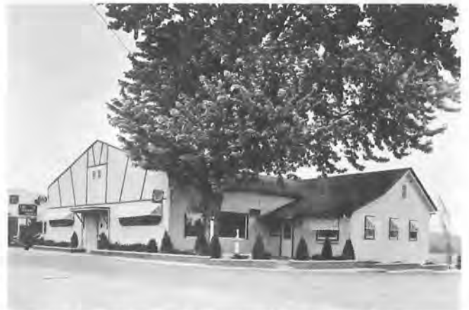
The Towne House as it appears today, on Merrill Avenue.
