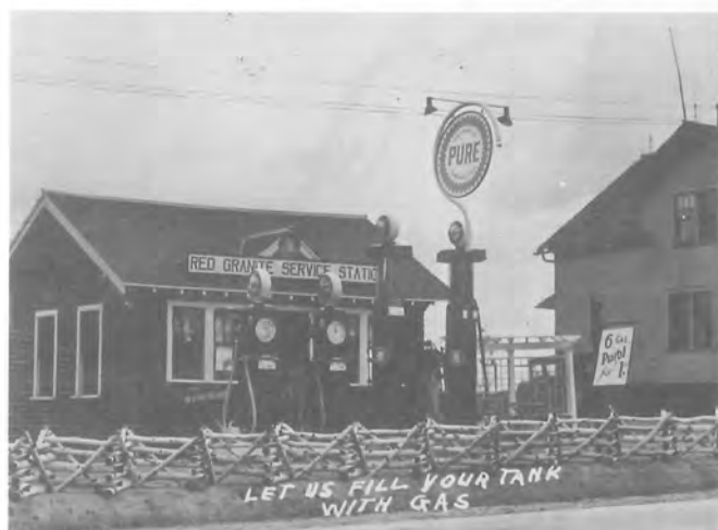
For the 6 gallon for $1.00, we could go back to the good old days. The Red Granite Service Station.
