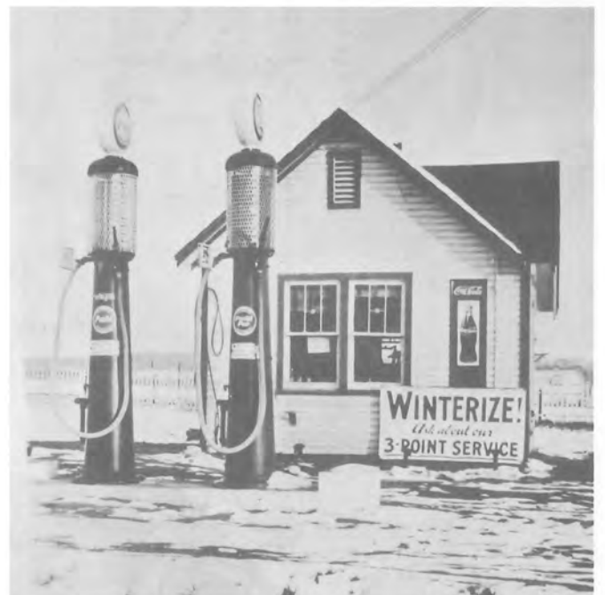
Reno Zastrow's filling station, on the corner of A and 51. Gas was pumped into the glass holding tank, where it was measured and then it was gravity fed into the gas tank.
