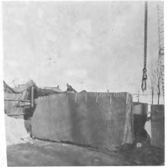
Largest stone ever taken out in the history of Rib Mountain Quarry. About 4,000 lb., 12 ft. 6 in. long, 5 ft. wide, 2 ft. 6 in. in height. Note the drill holes.
