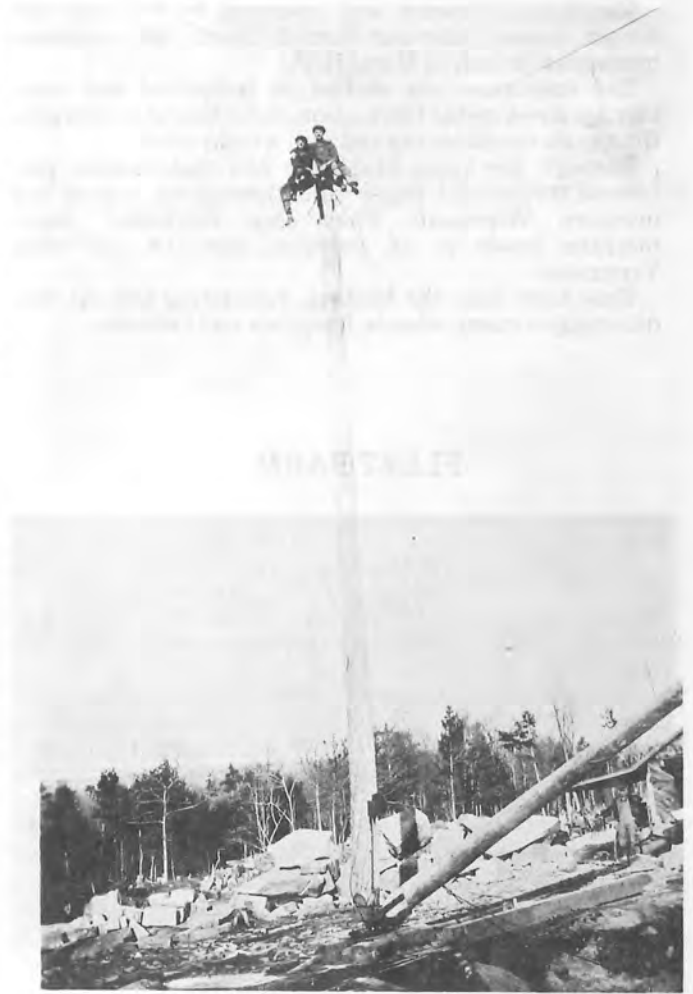
Edmund Woller and Arthur Sturm oiling the derrick.
