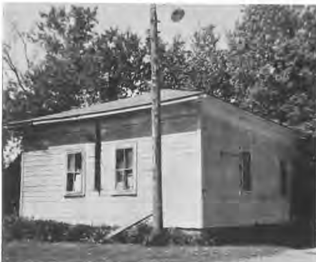
Building used for cheese making, still standing on the Otto Beilke farm, at 60th and Naught Drive.
