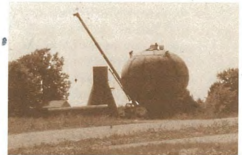
The new water tower under construction.
