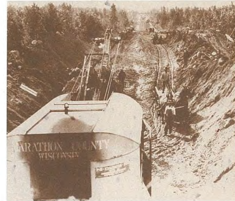
Building the road up Brokaw Hill.
