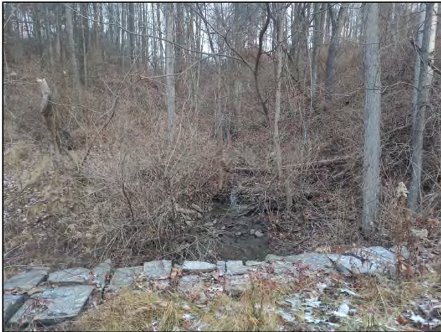
Photo 04. Photo showing the steep outfall of Stream 2 through a culvert outside of the delineation area, facing north.
