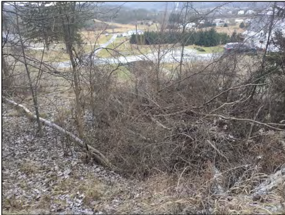
Photo 16. Photo showing the culvert outfall from Stream 2 as it drains under the road, showing the steep slope leading up to the property, facing south.
