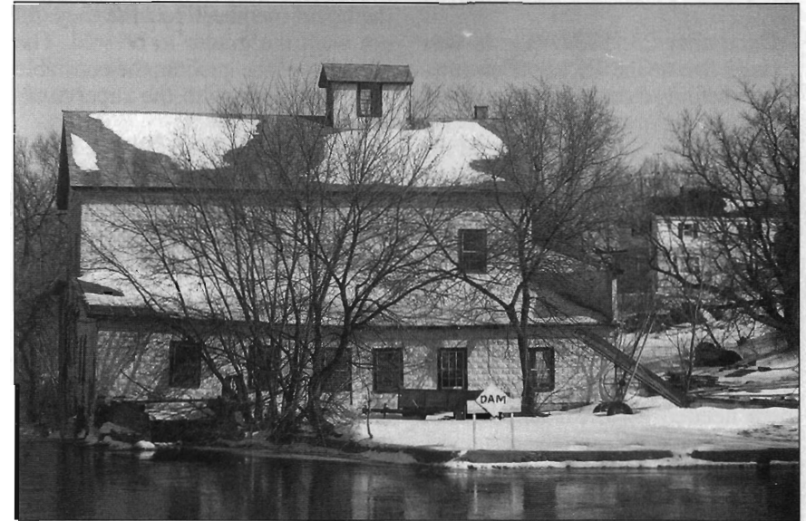
The historic Rockville Mill, dating back to 1914, was dismantled following the turn of the century to make way for improvements to the Rockville Dam as part of the millpond preservation effort. Originally built by the Meyer family, it was operated for many years by Willard Hahn.
