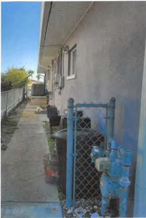
Side of house from the front
