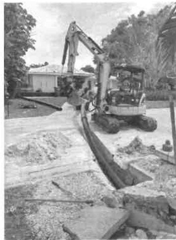
PIPE SLIP LINING AS NEEDED
