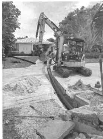
PIPE SLIP LINING AS NEEDED
