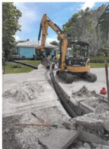
PIPE SLIP LINING AS NEEDED
