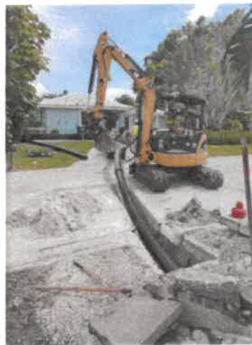
PIPE SLIP LINING AS NEEDED
