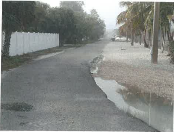
Palm Ave Before Construction 1/9/2018)
