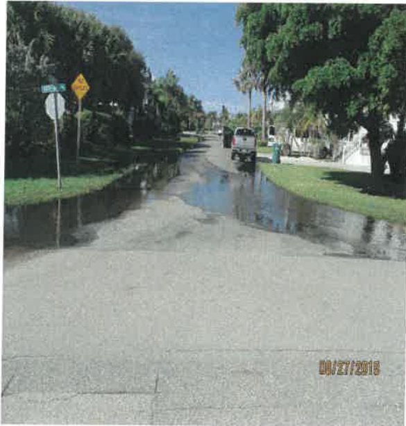
Kumquat at South Before Construction
