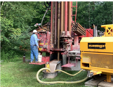
Above: Driller installing new private deep well
