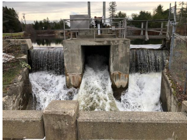
Figure D - 2: Toddy Pond Dam
