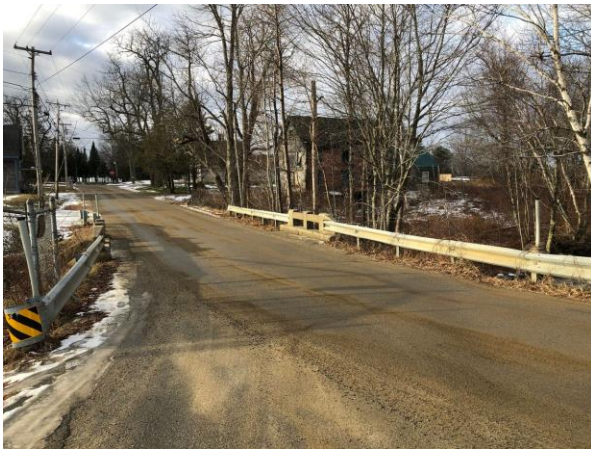
Figure D - 1: Image of Bridge over Toddy Stream
