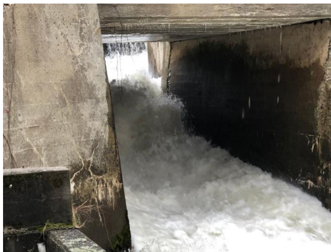
Figure D - 3: Bridge Substructure at Toddy Pond Dam .
