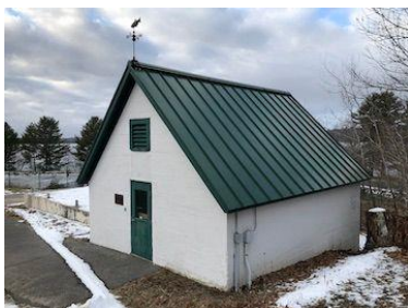
Ice House (1896), only remaining structure of original Craig Brook National Fish Hatchery, the first salmon hatchery in the United States, started in 1871 by Maine, Massachusetts, and Connecticut, designated a federal hatchery in 1989.
