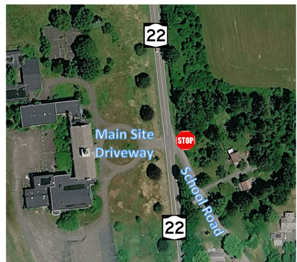
Aerial Photo #2 – NY Route 22/School Road/Driveway
