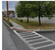
ADA Compliant Curb Ramps with detectable warning units
