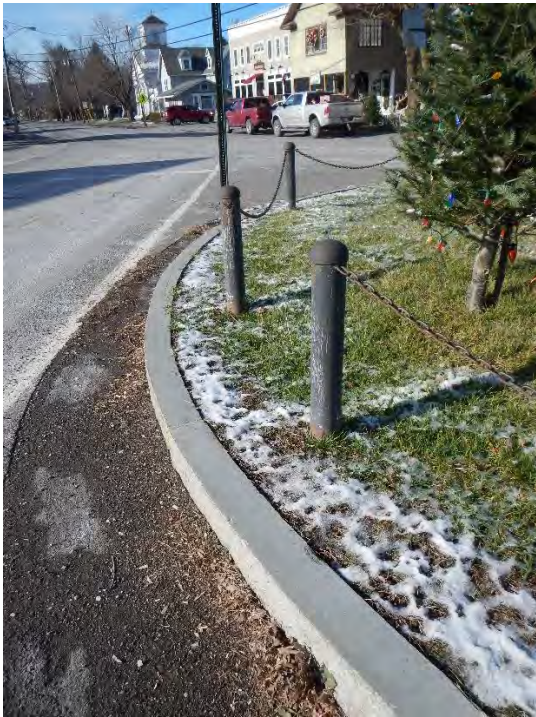
Figure B-9 - Close-up photo of granite curb, metal bollard, and connecting chain.
