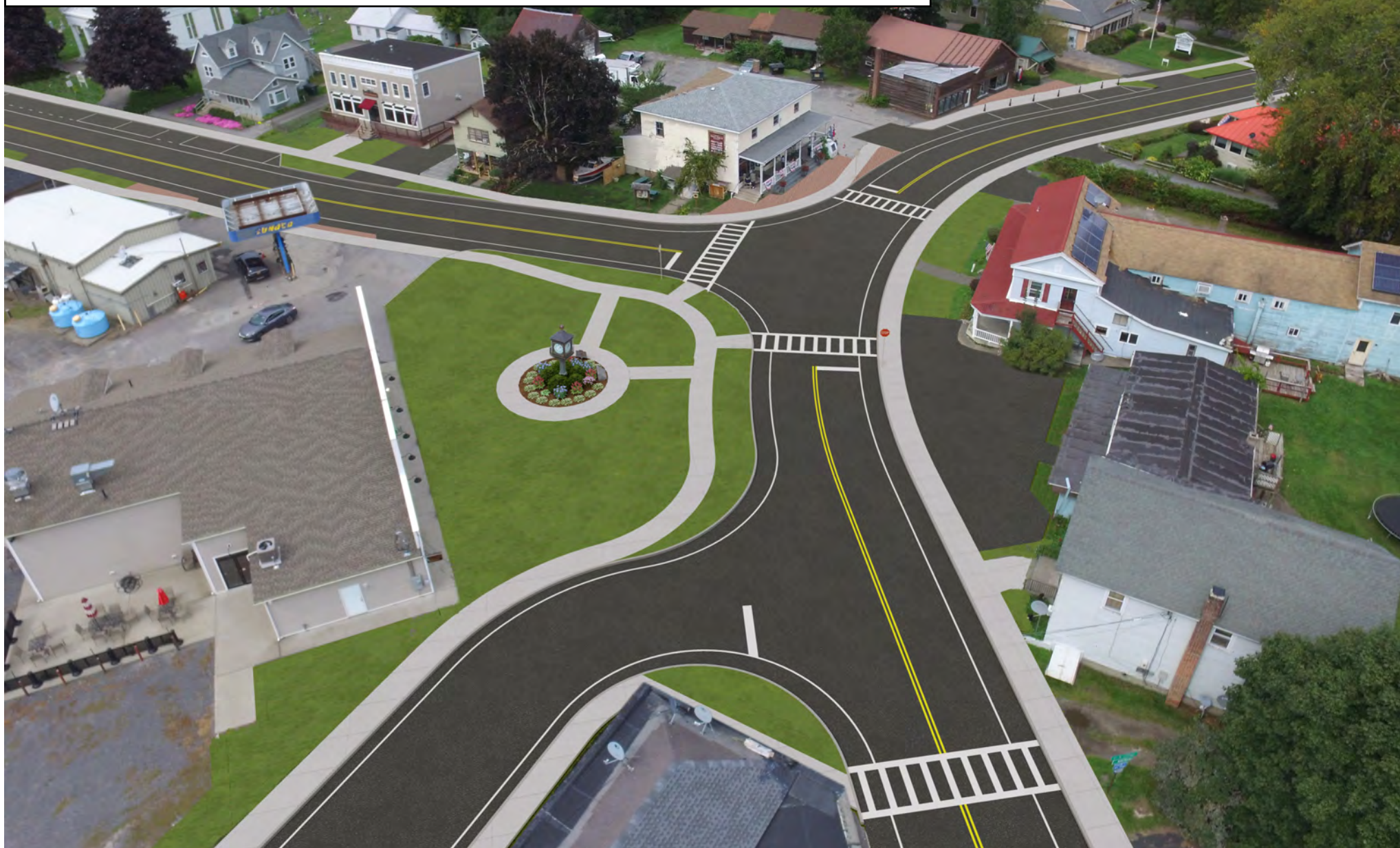
Figure C-6: T-Intersection with Clock Relocation Alternative Rendering (Preferred Alternative)
