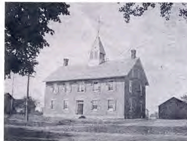
Chazy Village school from 1874 until 1916—it is now the front part of Gray Gables.
