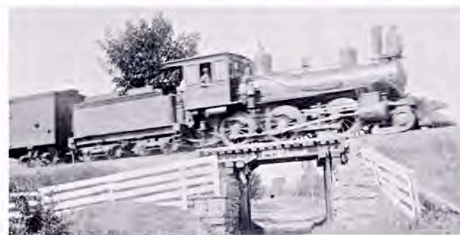
Clark Street railroad overpass.
