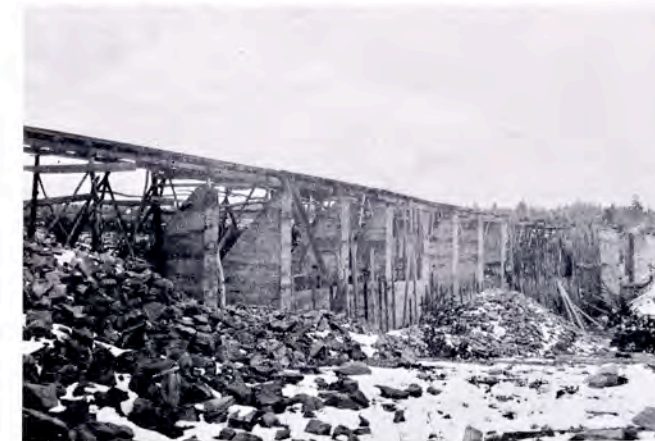
The "Million Dollar Dam" under construction.
