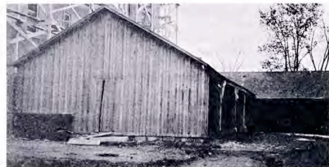
The Chazy Methodist Church sheds in October 1920 with Gray Gables under construction behind them.
