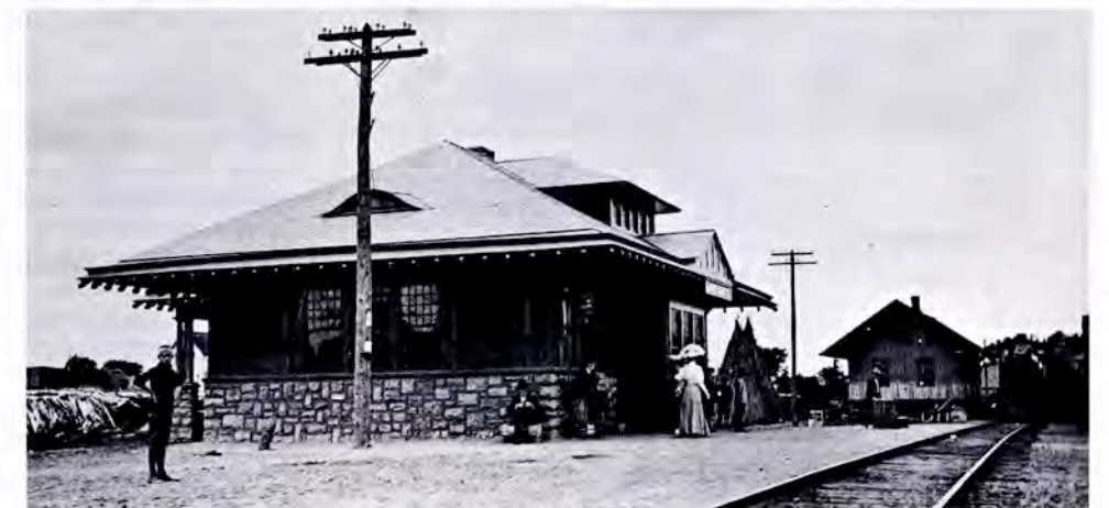
The West Chazy stations—the first station is to the rear.
