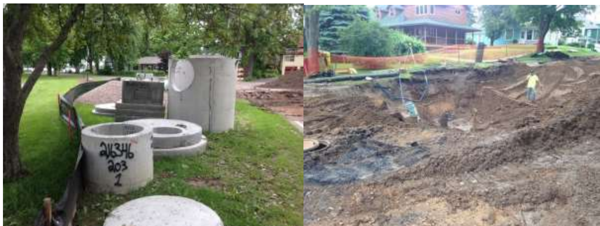
Figure 33: Humbird Street Grit Chamber Installation
