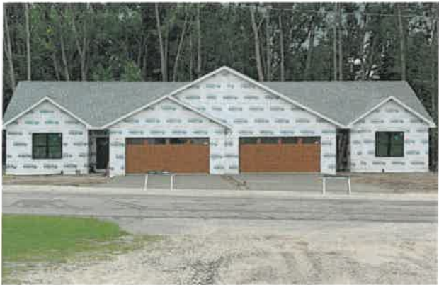
New twinhome construction in Pelican Rapids
