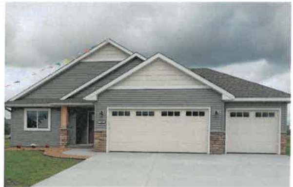
1 Level Home in Sauk Rapids Constructed by DG Homes
