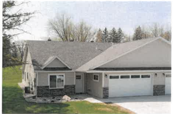
Twin Home in Fergus Falls Constructed by Rogness Contracting
