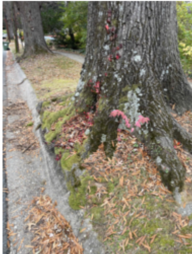
Large shade trees in small planting areas lead to infrastructure issues
