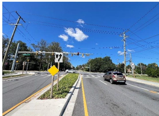
Photo 3 - WB Jones Bridge Rd
