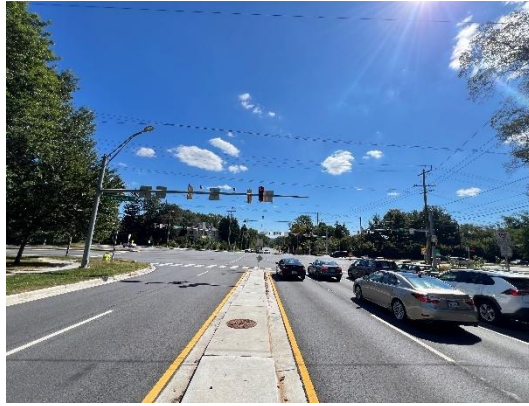
Photo 4 - EB Jones Bridge Rd
