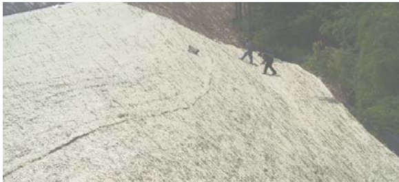
Example of a maximum 3:1 slope
