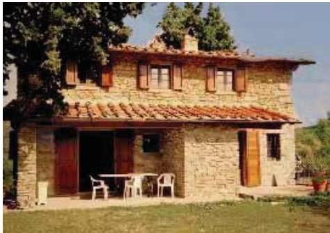
(Image 112a) Exterior wall with projections & recesses
