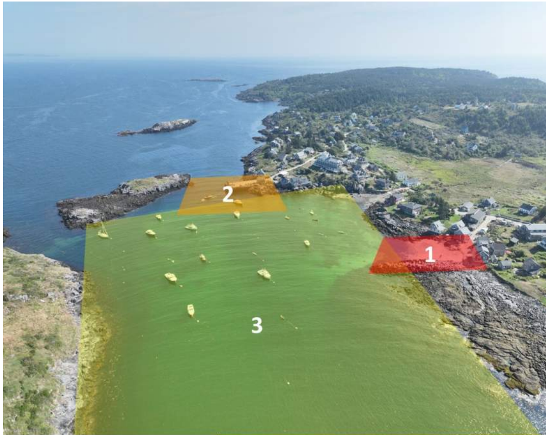
Figure 1-2. Aerial Image of Monhegan Harbor Looking North, with the Three Areas Targeted for Study of Improved Wave Protection.
