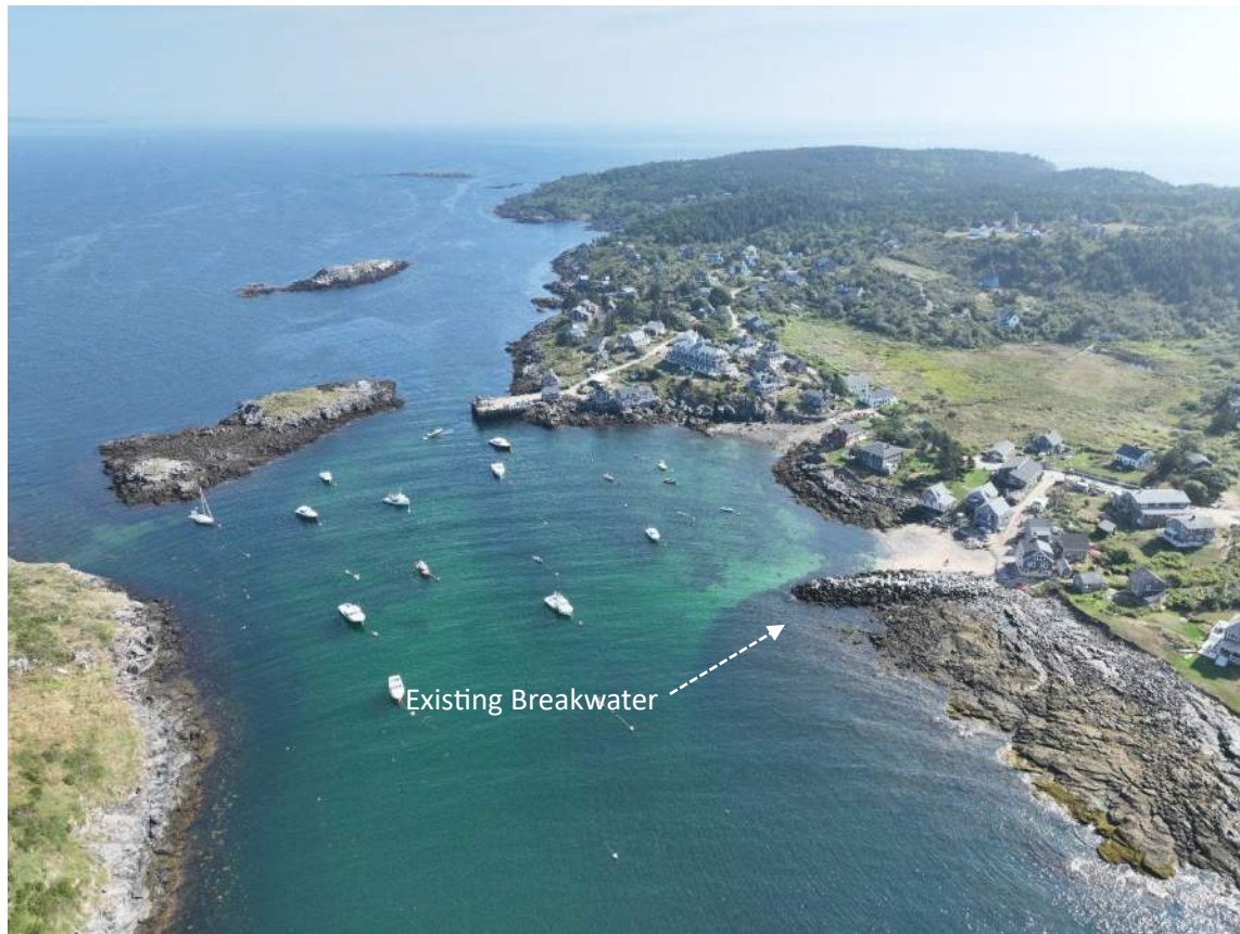
Figure 1-1. Aerial image of Monhegan Harbor Looking North.
