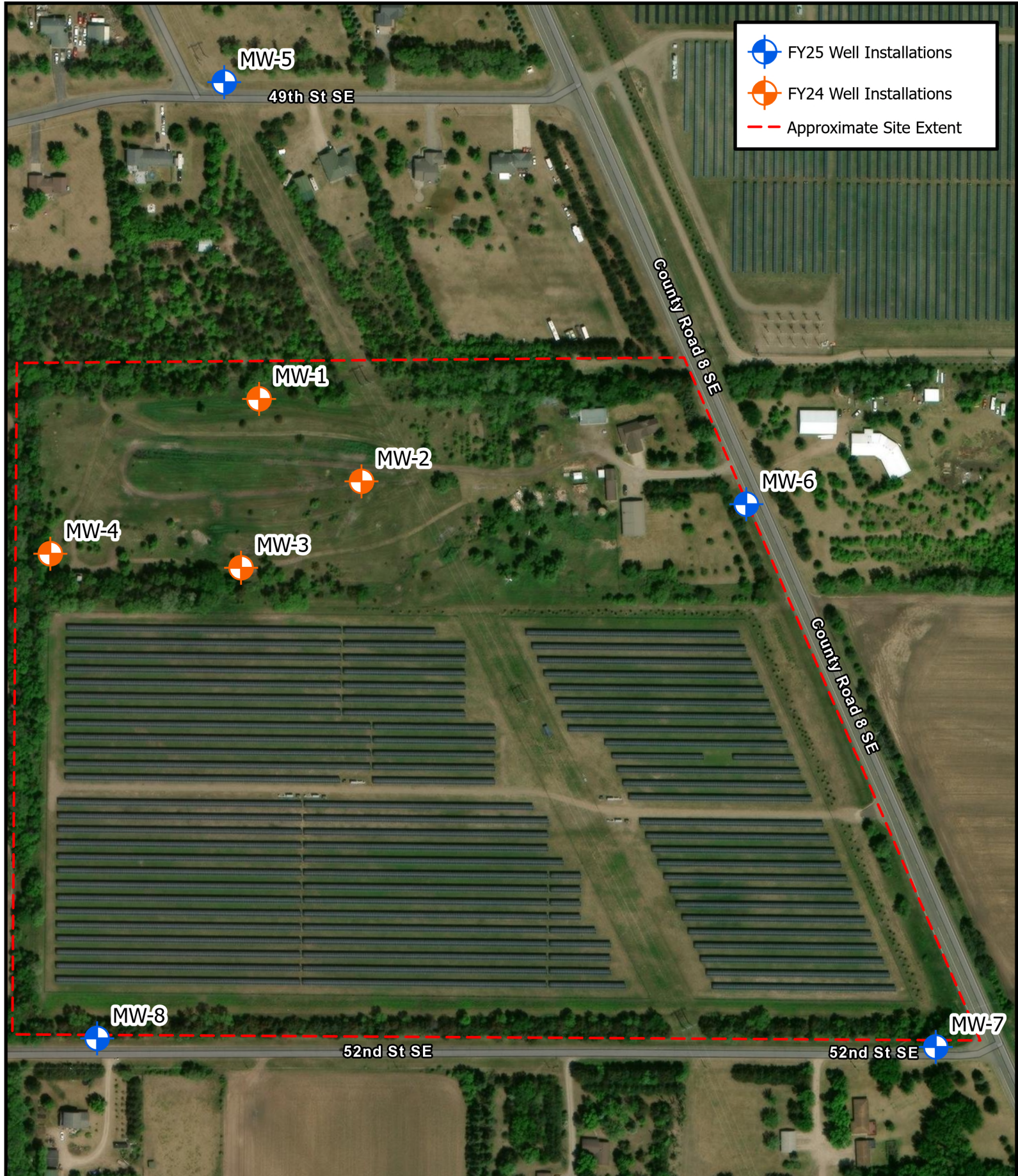
Figure 1 Wells Installed in FY24 and FY25 St. Cloud PFAS Forensics Minnesota Pollution Control Agency
