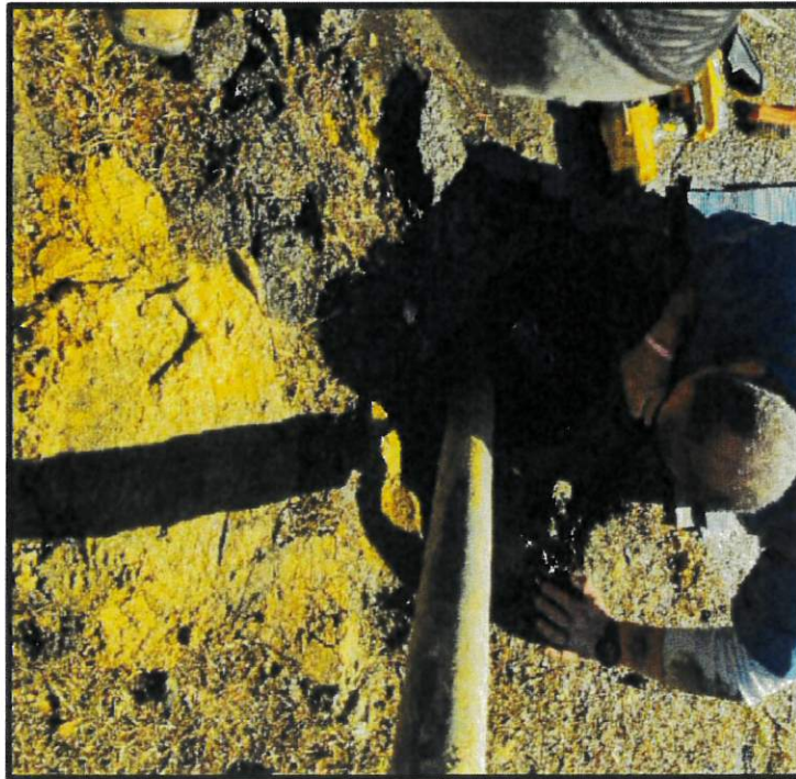
Figure 1 – David Street Leak Repair
