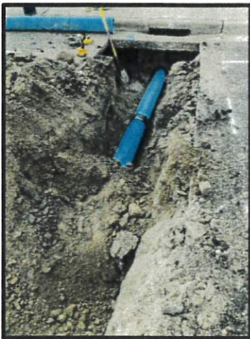
Figure 1 - Stormwater Pipe Replacement Pine Street
