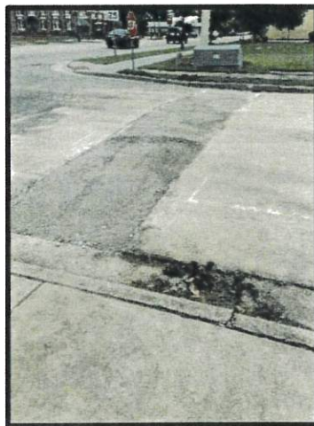
Figure 2 - Stormwater Pipe Replacement Pine Street After
