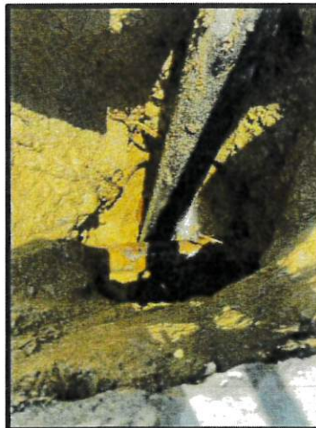
Figure 3 - 2" Water Leak
