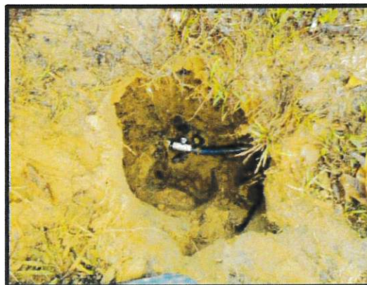
Figure 1 - Leak Repair @ Lower Street
