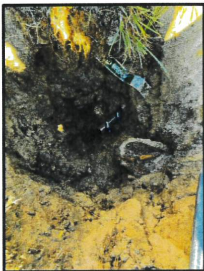
Figure 2 - Leak Repair 119 Courthouse Drive
