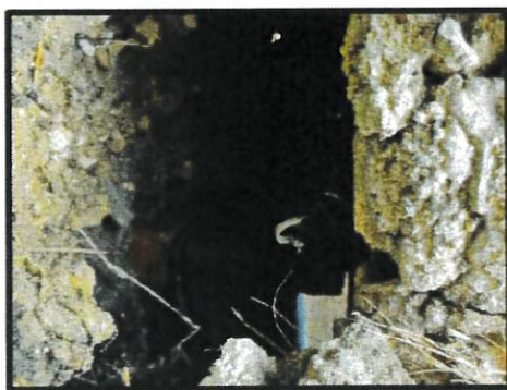
Figure 2 - S Lower & King Storm Repair
