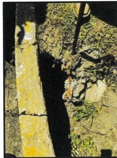
Figure 1 - S Lower & King Storm Repair
