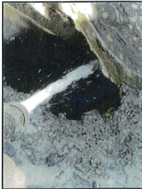
Figure 2 Martin Luther King, Jr. Leak Repair
