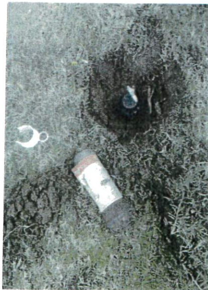
Figure 2 Replacing Sprinkler Heads
