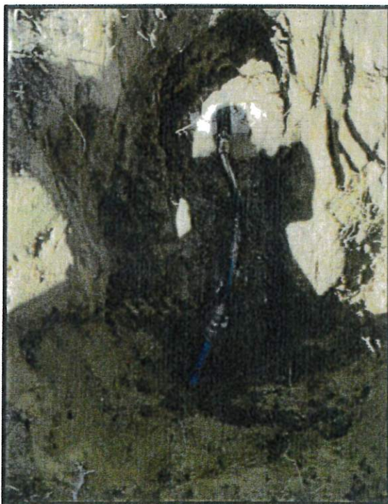
Figure 1 Brisson Street Leak Repair
