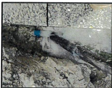
Figure 3 Mill Street Before & After
