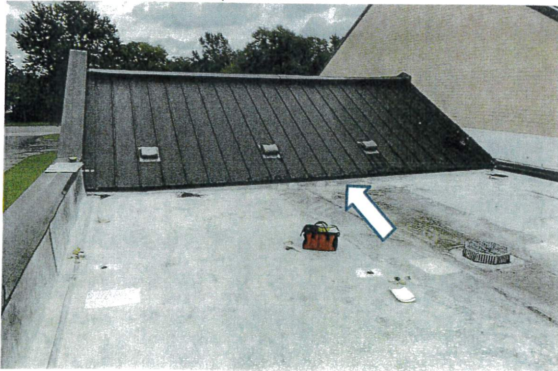
Photo 4 – View of limited flashing height conditions at transition between the standing seam metal roofs and the low sloped roof areas.
