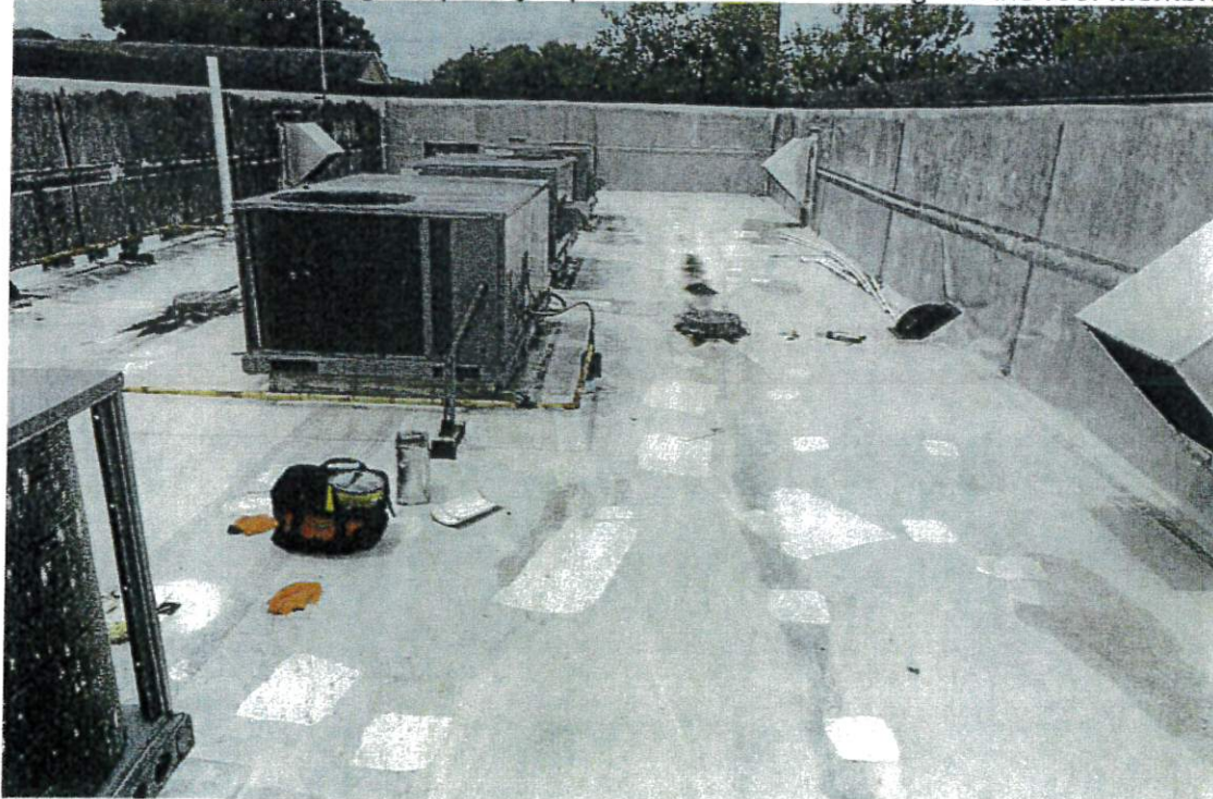
Photo 6 – Photo showing temporary repairs at hail strike damage to the roof membrane
