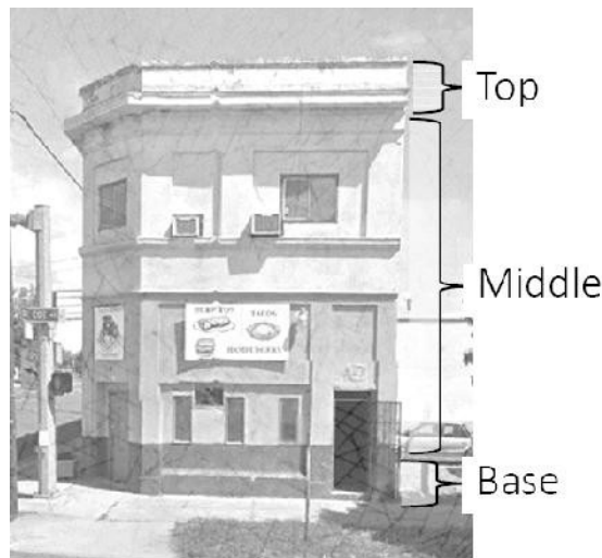
Figure 2.2.160B(3) –Building Base, Middle and Top
